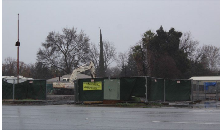
Oleander Community Housing Apartments, Esplanade, Chico – Construction start, Underground
