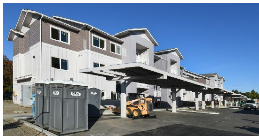
Woodward Family Apartments, 263 Swift Street, Orland
