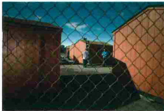
City is building modular structures for its first sanctioned homeless encampment on 6th and Brush on 12-04-17, Oakland, California. Photo by Paul Kuroda
