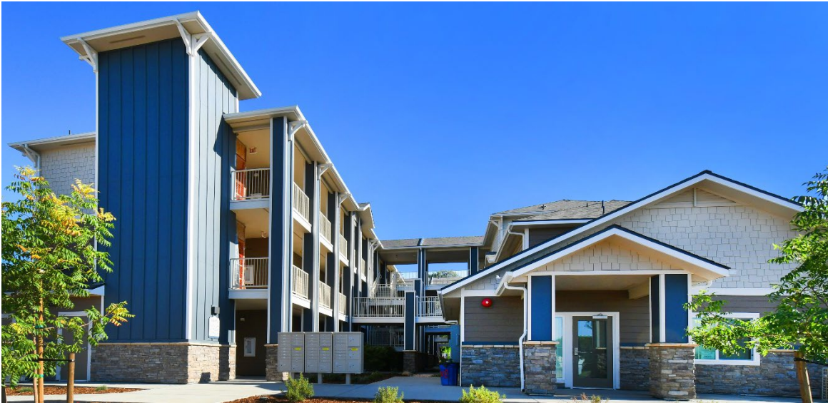
Mitchell Avenue Apartments II, Mitchell Avenue, Oroville
