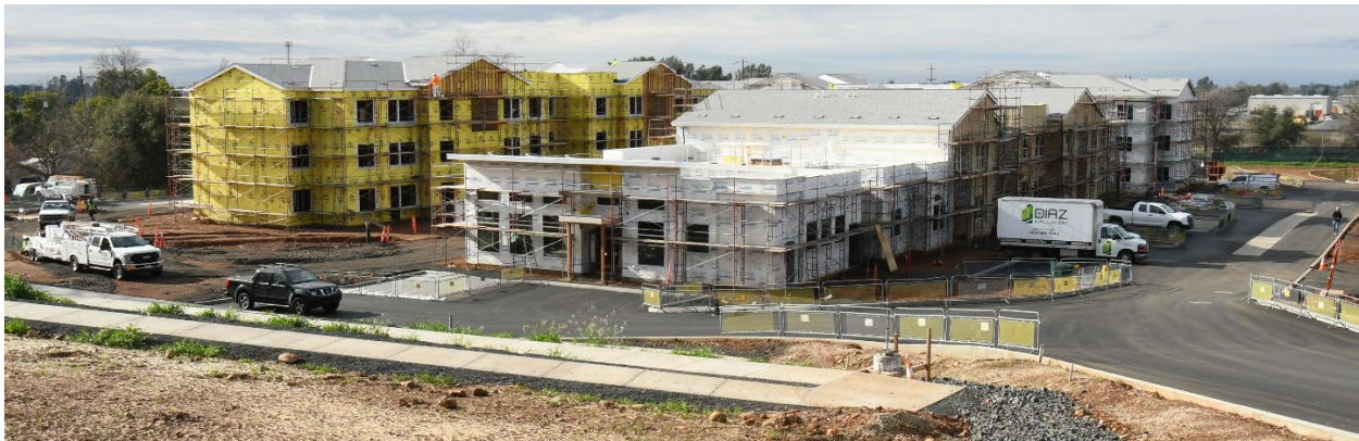
Lincoln Family Apts, 3300 Lincoln Boulevard, Oroville
