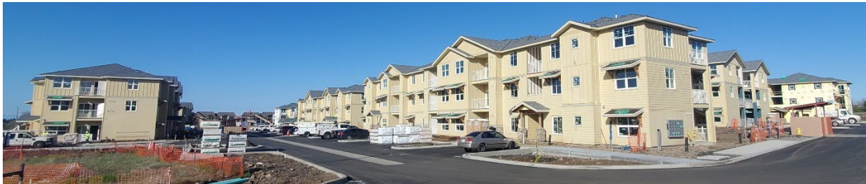
Deer Creek Apartments I & II, Highway 32, Chico
