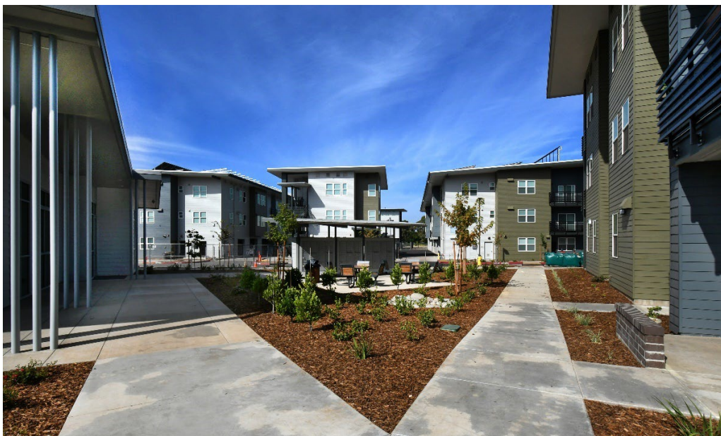
North Creek Crossings Apartments I, Meriam Park, Chico
