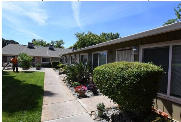
Park Place Apartments, 2105 Park Avenue, Oroville
