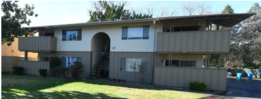
Cordillera Apartments, Cameo Way, Chico
