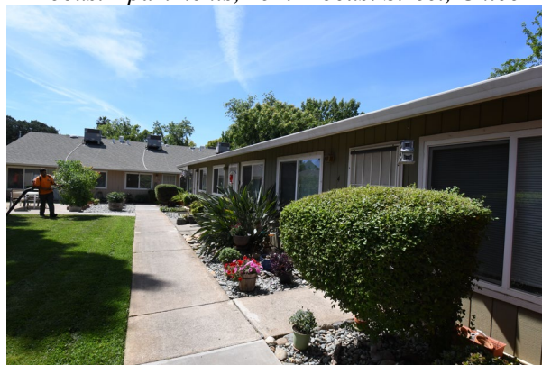
Park Place Apartments, 2105 Park Avenue, Oroville
