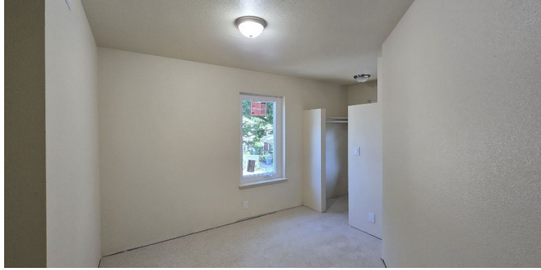
645 Gardella Avenue, Oroville (rehabilitation in process)
