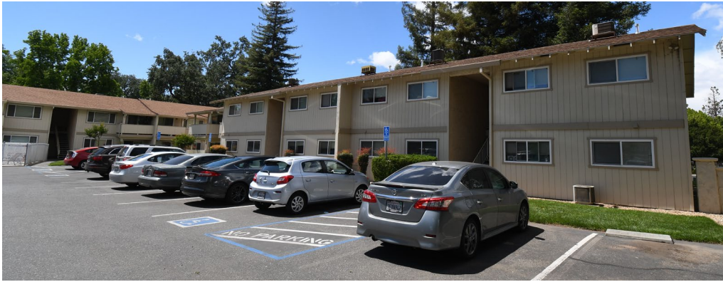
Alamont Apartments, 811 West East Avenue, Chico
