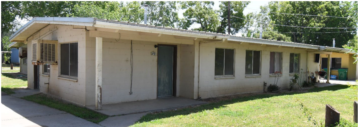
Unrenovated 1980's era Concrete-block Unit
