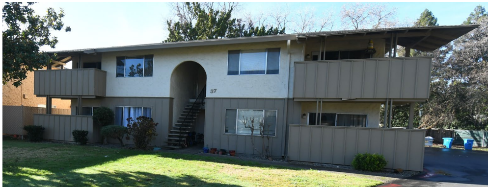
Cordillera Apartments, Cameo Way, Chico
