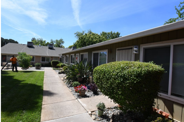
Park Place Apartments, 2105 Park Avenue, Oroville
