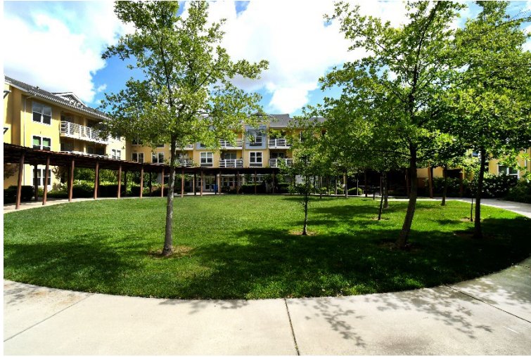
1200 Park Avenue Apartments, Inner Courtyard view
