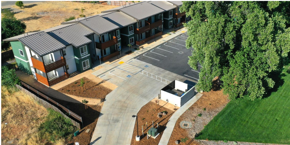
Photo of completed project
