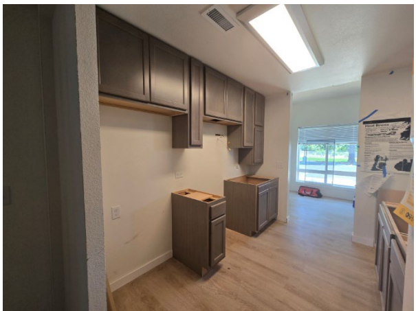
New cabinet installation in process
