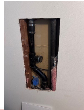
Drainpipe Repair Build. #41
