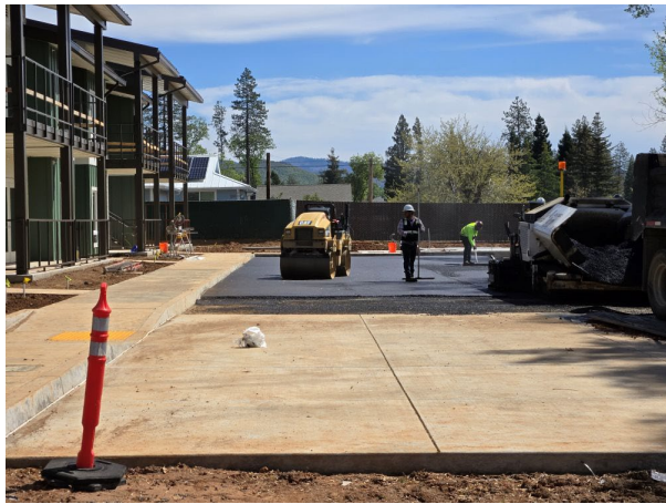
Parking lot asphalt overlay in process
