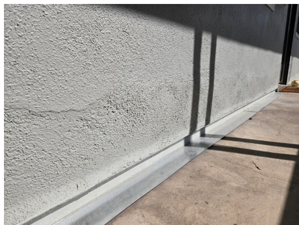
Stucco patch, flashing and paint match complete
