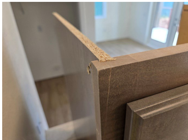
Photo of cabinet with damage and MDF sides
