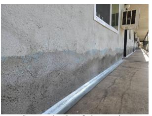
Stucco patch and new flashing complete
