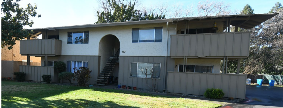
Cordillera Apartments, Cameo Way, Chico
