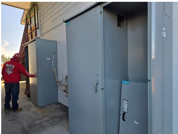
Electrical switchgear installation in progress
