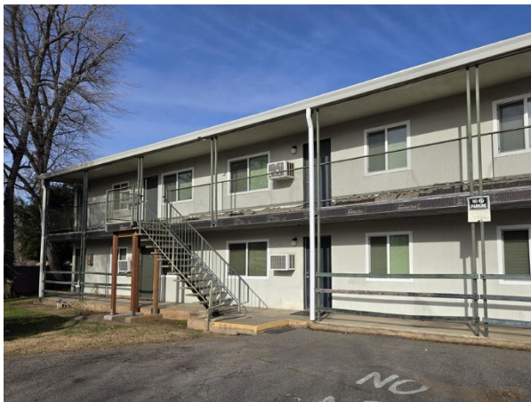
Stucco lath in progress
