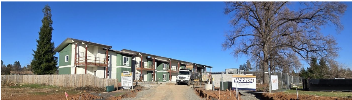
Photo of overall construction progress
