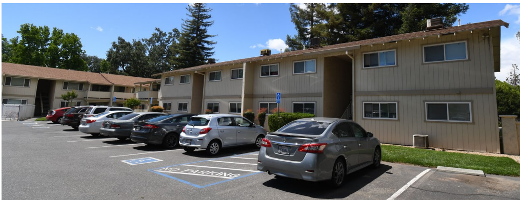
Alamont Apartments, 811 West East Avenue, Chico
