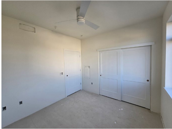
Typical interior bedroom progress
