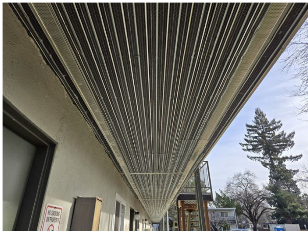
Plaster lath in progress
