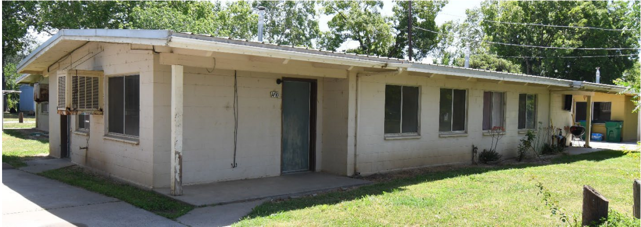
Unrenovated 1980's era Concrete-block Unit
