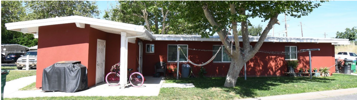
Renovated 1980’s era Concrete Block Housing
