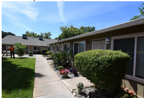
Park Place Apartments, 2105 Park Avenue, Oroville
