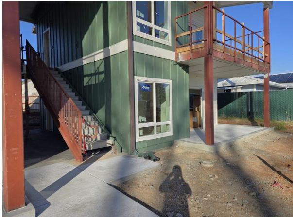
Site concrete installation in progress
