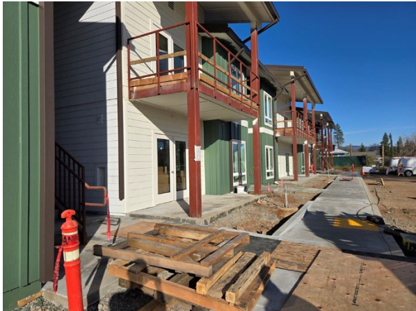
Site concrete installation in progress
