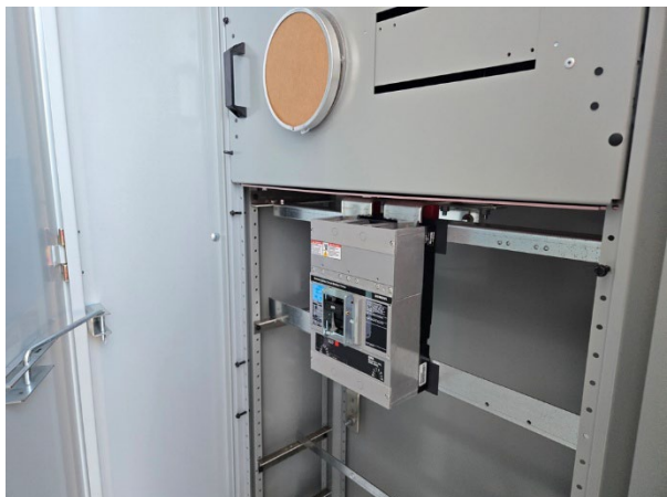
Electrical switchgear installation in progress
