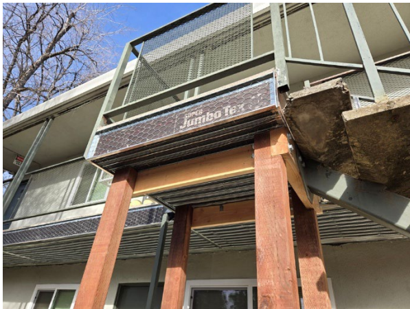
Stair landing reconstruction nearly complete
