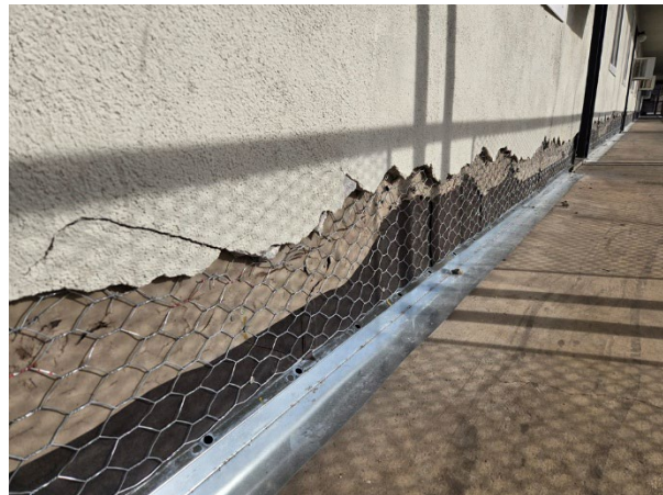
Stucco lath and new metal flashing in progress
