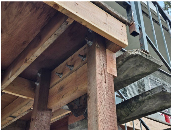
Stair landing reconstruction nearly complete
