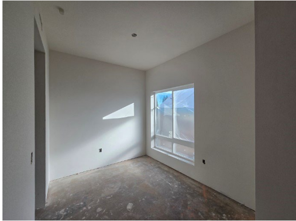
Drywall texture application complete
