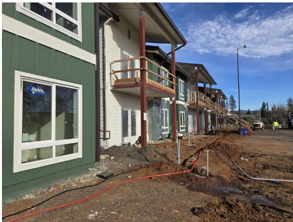
Exterior painting nearly complete
