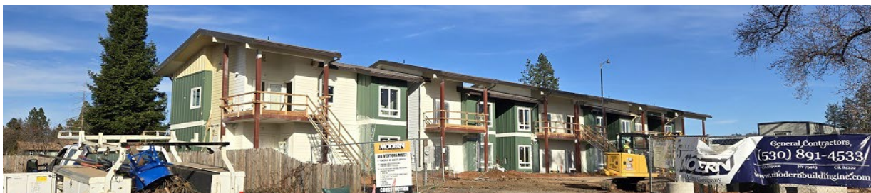
Photo of overall construction progress
