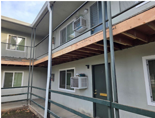
Wood joist repairs complete
