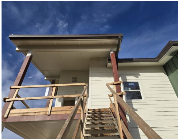
Exterior painting nearly complete
