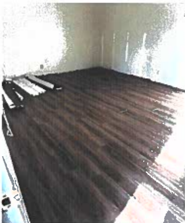
New flooring unit #11
