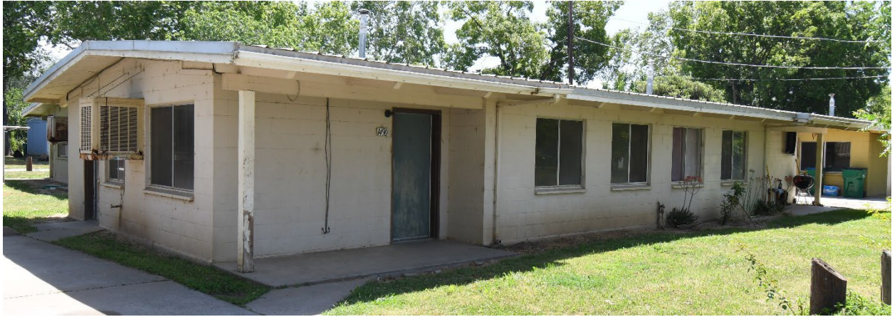
Unrenovated 1980's era Concrete-block Unit
