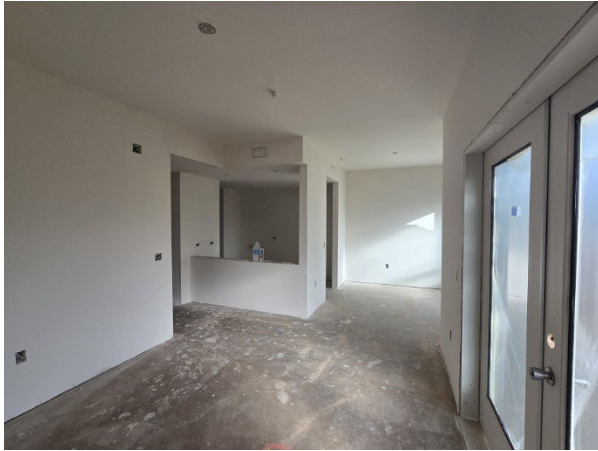
Drywall texture application complete
