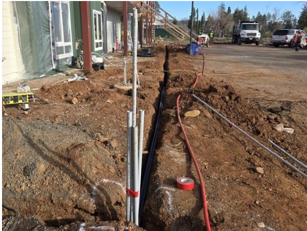
Site lighting infrastructure in progress
