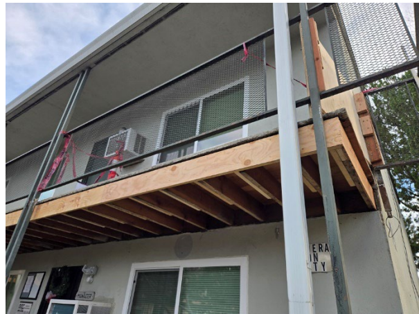
Wood joist repairs complete
