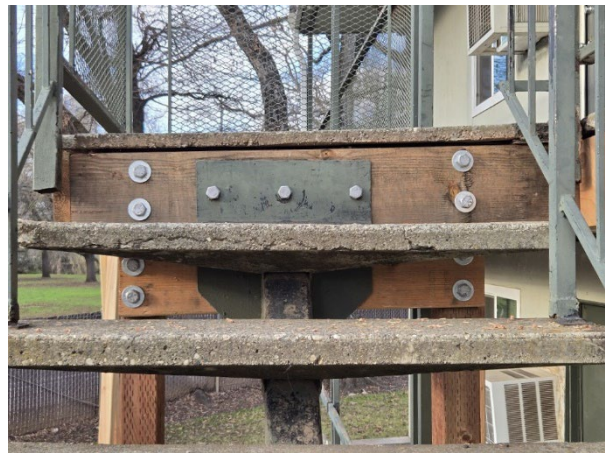
Stair landing reconstruction nearly complete
