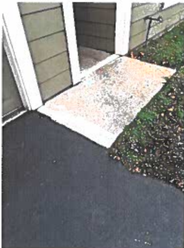
CONCRETE GRINDING
