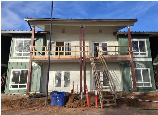
Exterior painting nearly complete
