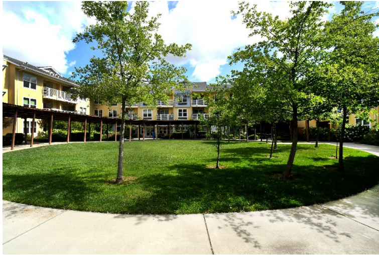
1200 Park Avenue Apartments, Inner Courtyard view
