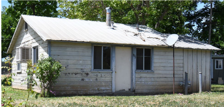
1930's era Wood Frame Units
