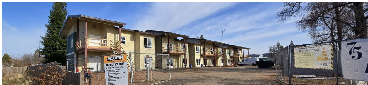
Photo of overall construction progress
