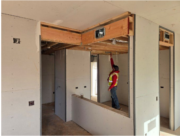
Drop ceiling framing complete
