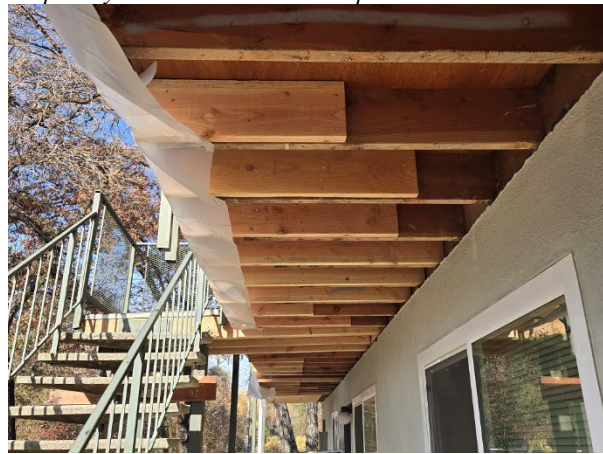
Wood joist repair nearly complete
