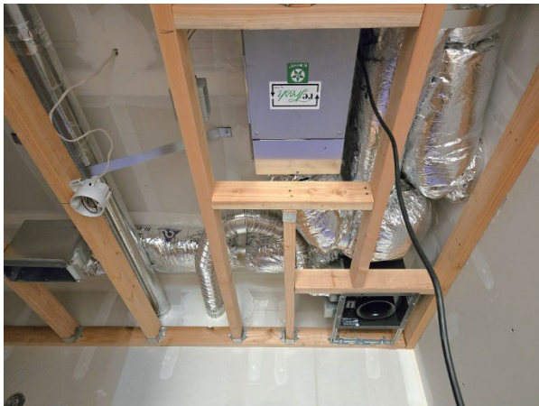
Heat pump HVAC rough-in complete
