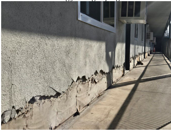
Stucco removed at second level for new waterproofing
