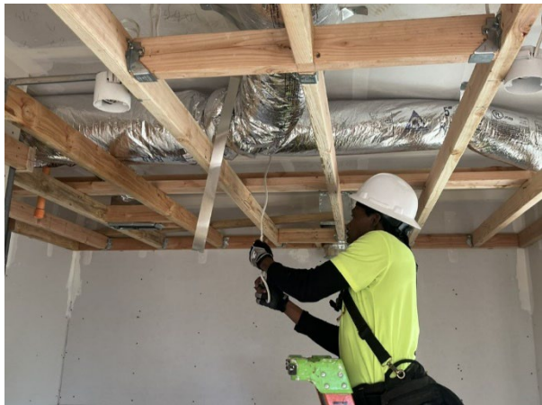
Heat pump HVAC rough-in complete
