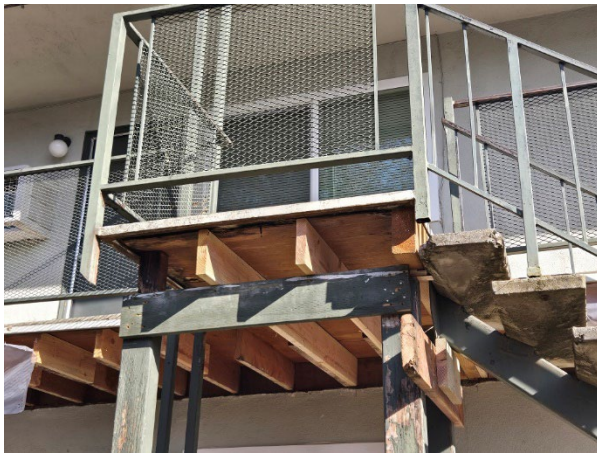
Stair landing framing in progress
