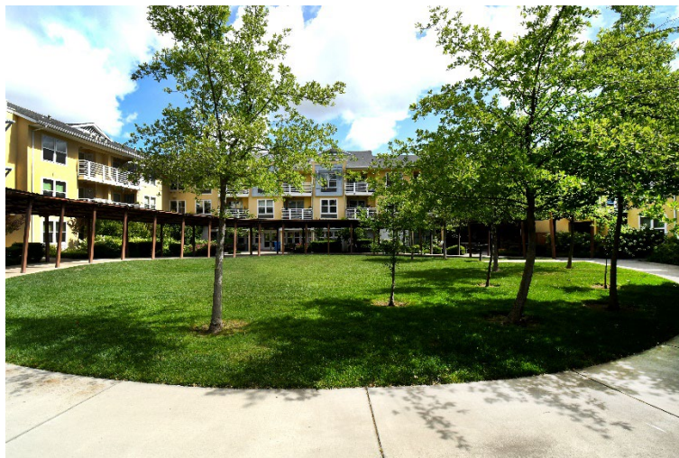
1200 Park Avenue Apartments, Inner Courtyard view
