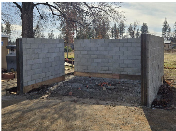
Cement block trash enclosure nearly complete
