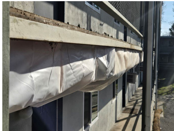
Temporary measures installed to prevent water intrusion
