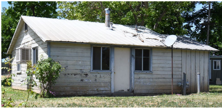
1930's era Wood Frame Units
