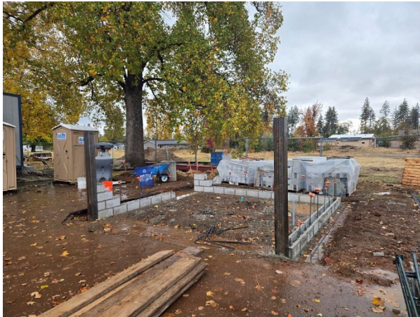
Cement block trash enclosure in process
