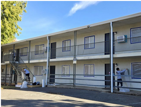
Preparation for demolition in process
