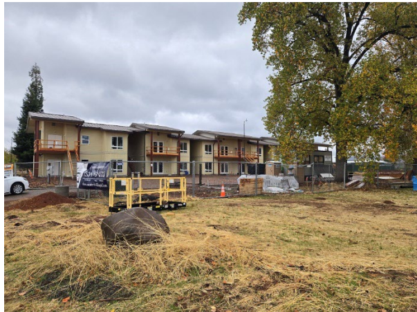
Siding and roof installation complete
