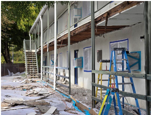
Demolition in process
