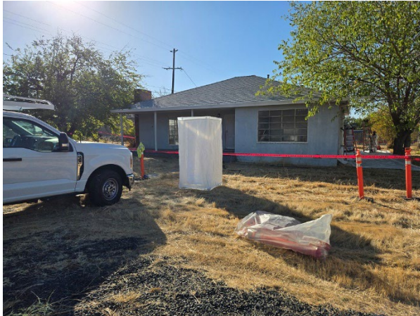
Asbestos and lead paint abatement in process
