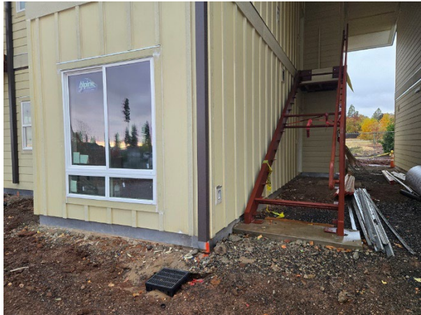
Siding complete and steel stair stringer in place
