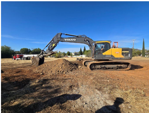
Demolition in process
