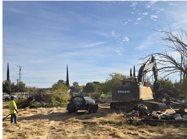
Demolition in process
