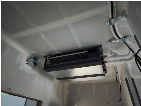
Heat pump HVAC system installation in process
