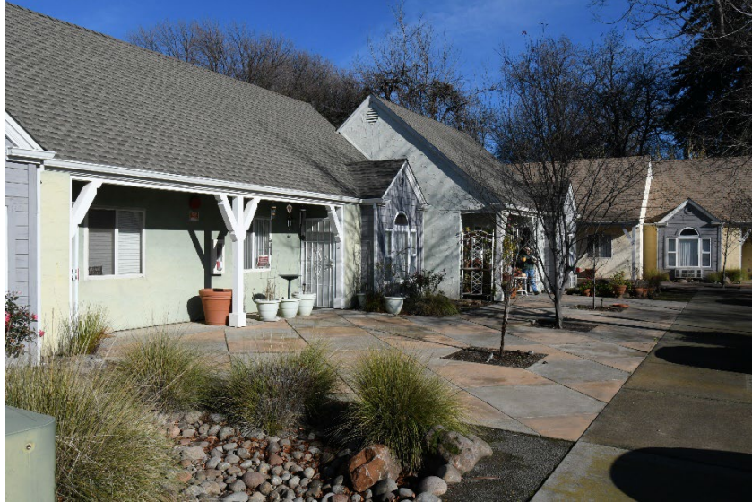
Walker Commons Apartments, 678 Buttonwillow Lane, Chico
