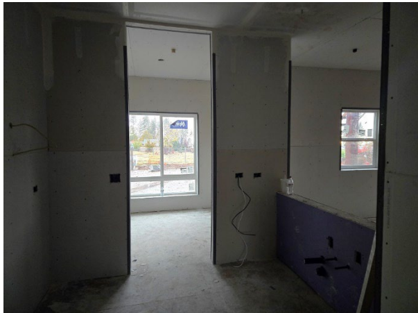
Drywall hung throughout all units
