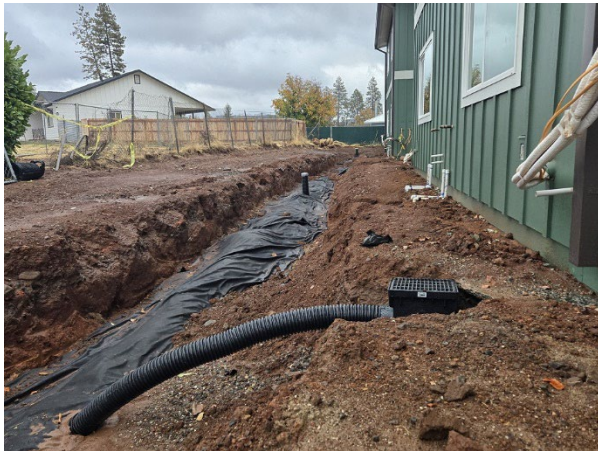
Drainage swale installation in process
