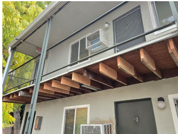
Demolition complete and repairs in process
