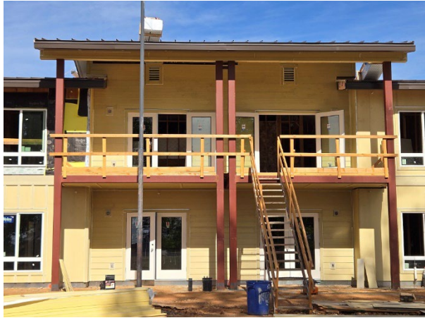
Siding installation at front of building
