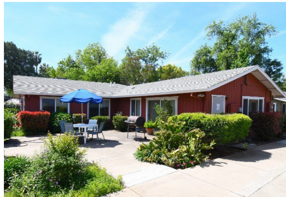
Community Building prior to improvements
