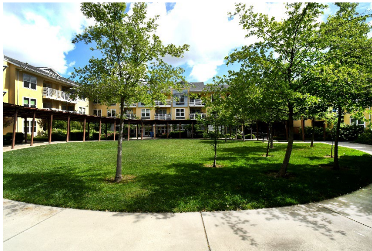
1200 Park Avenue Apartments, Inner Courtyard view
