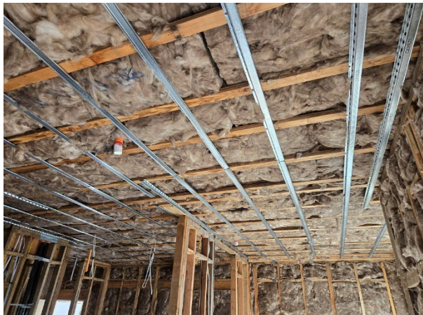
Sound dampening measures in place at first floor units
