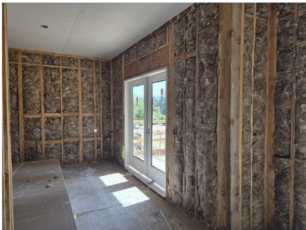
Insulation installed and drywall in process
