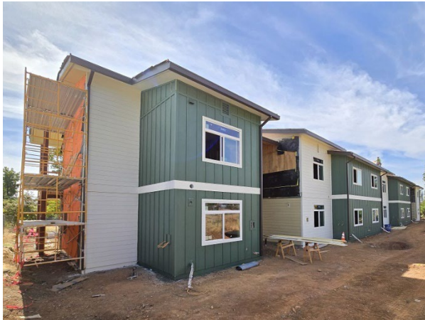
Exterior Painting at rear of building
