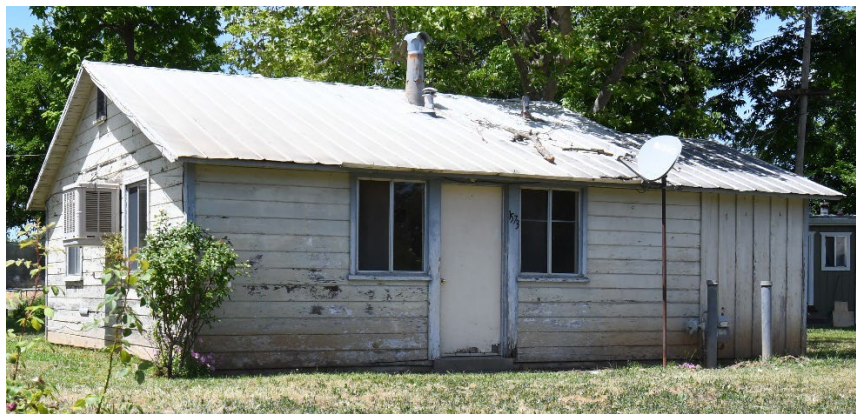
1930's era Wood Frame Units
