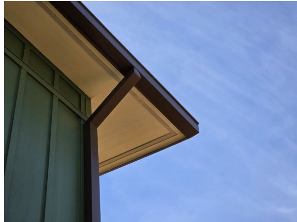
Soffits, gutters and downspouts installed
