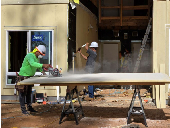
Siding installation at front of building
