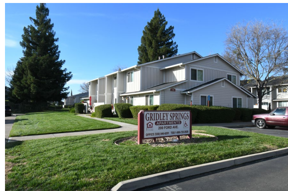
Gridley Springs Apartments II, 210 Ford Avenue, Gridley
