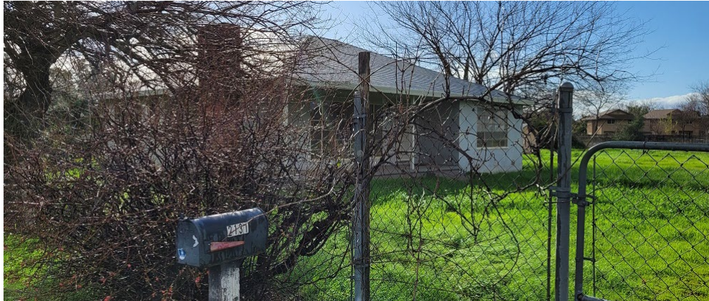
2131 Fogg Avenue, Oroville - Project site and structure slated for demolition
