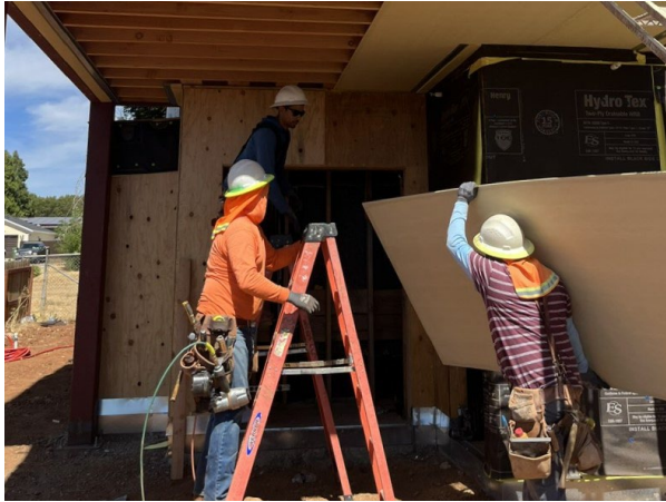
Soffit installation in process
