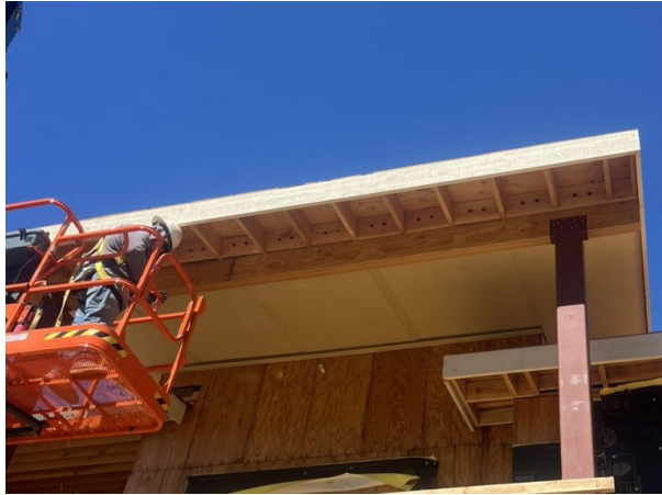
Soffit installation in process
