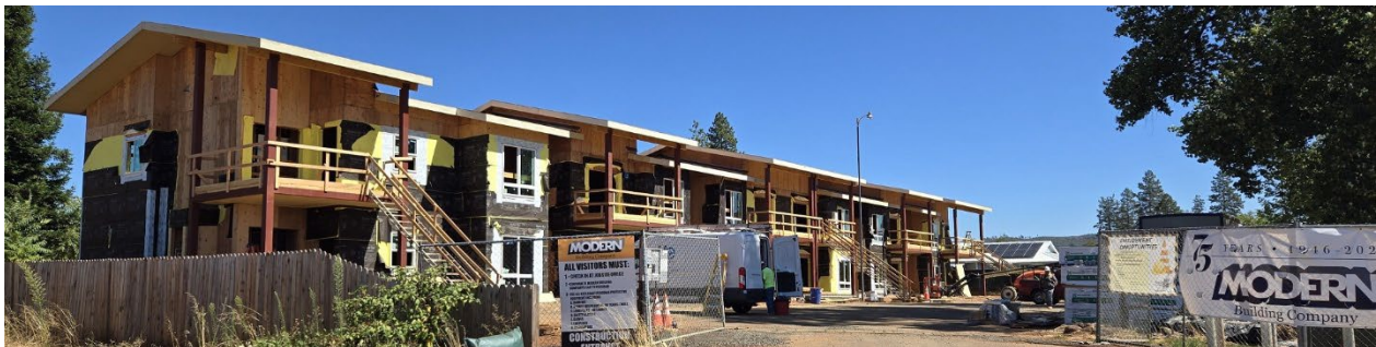
Photo of construction progress
