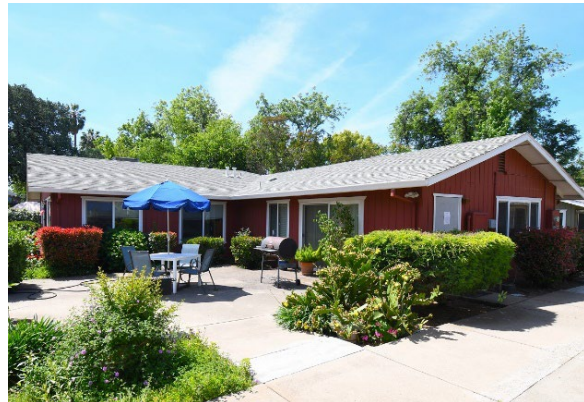
Community Building prior to improvements
