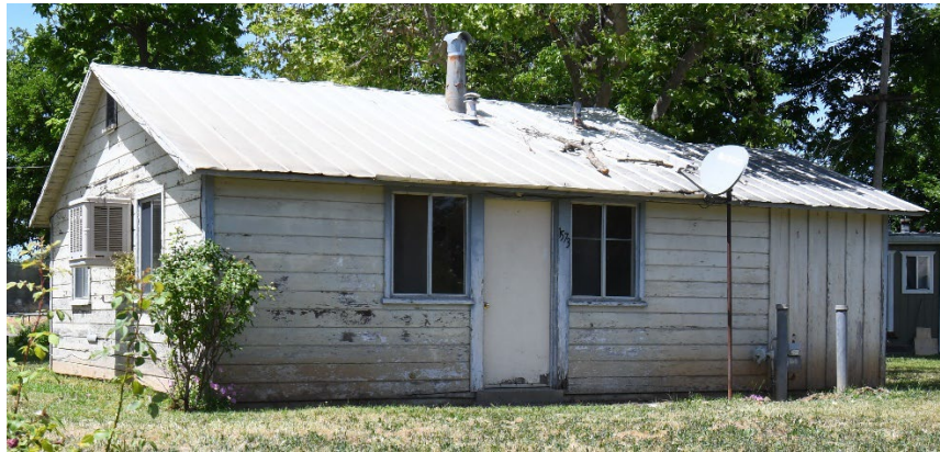
1930's era Wood Frame Units
