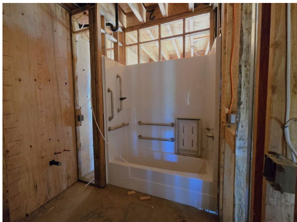
Tub inserts installed throughout
