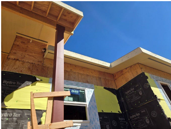
Enclosed eaves with fire-resistant venting
