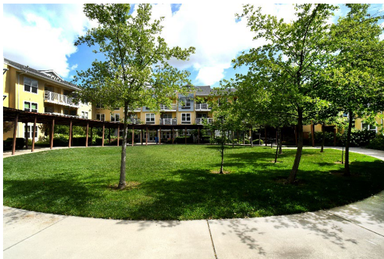
1200 Park Avenue Apartments, Inner Courtyard view
