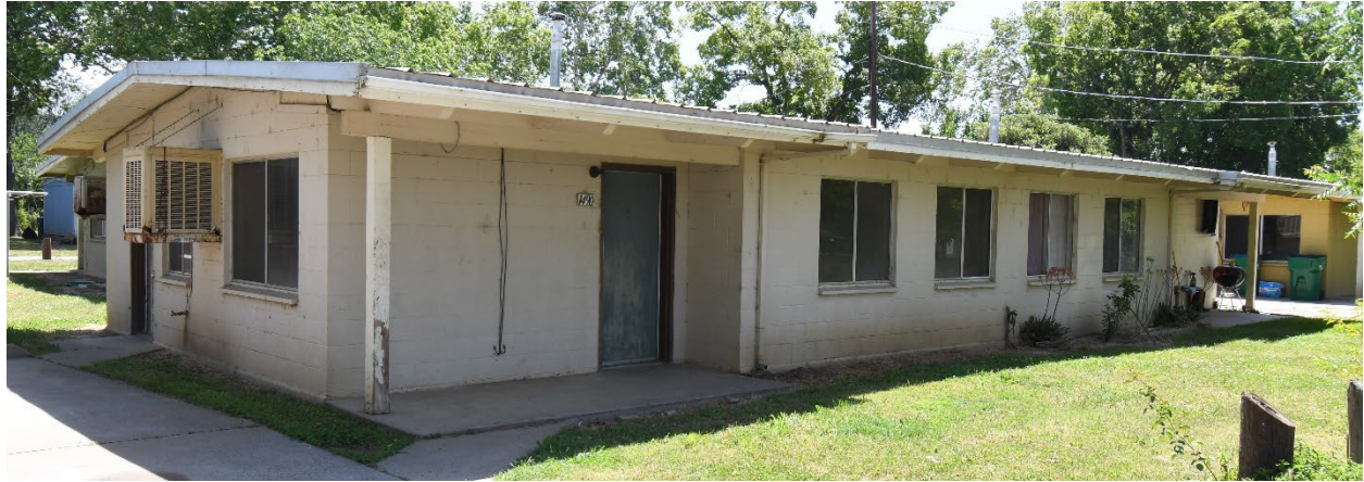
Unrenovated 1980’s era Concrete-block Unit
