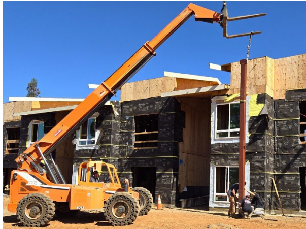
Structural steel installation
