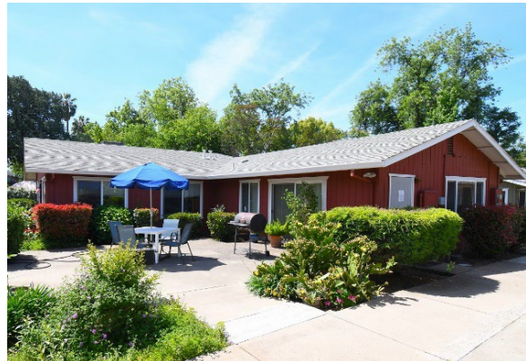
Community Building prior to improvements
