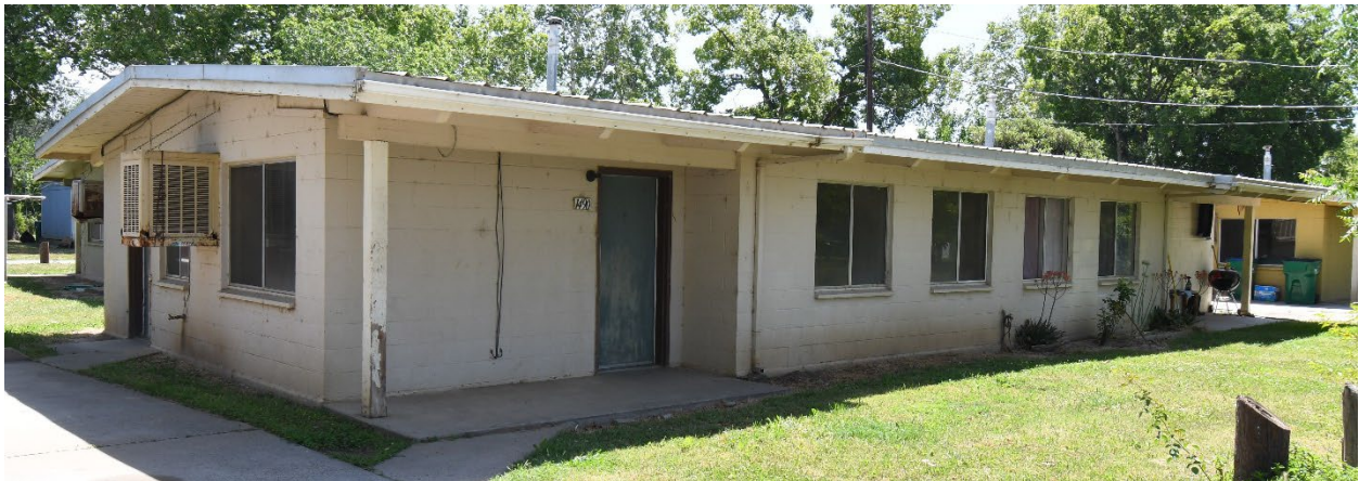
Unrenovated 1980's era Concrete-block Unit
