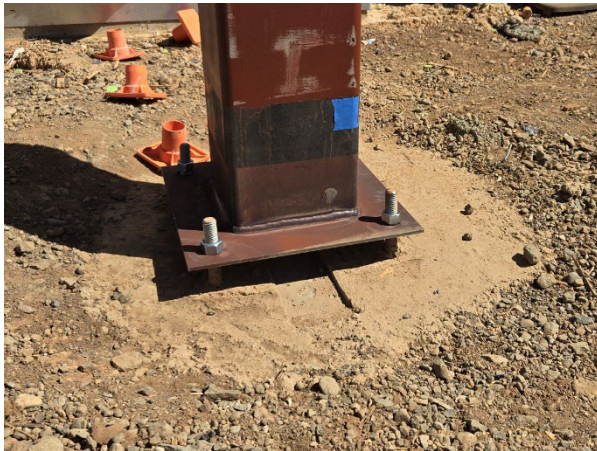
Structural steel base plate installation
