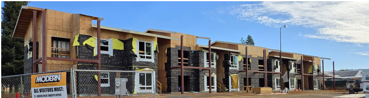
Photo of construction progress
