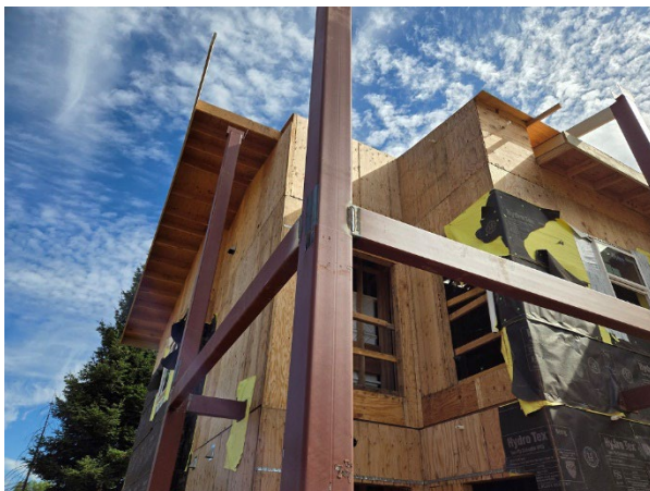
Structural steel installation complete
