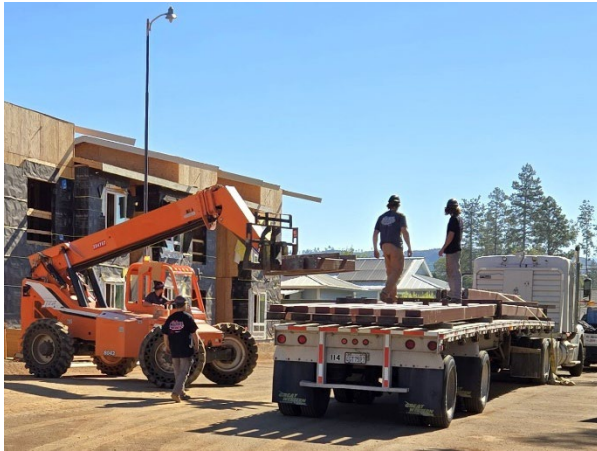
Structural steel delivery
