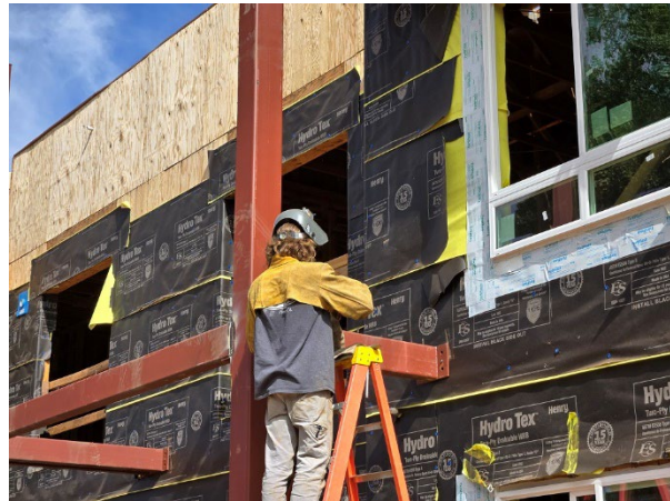
Structural steel welding
