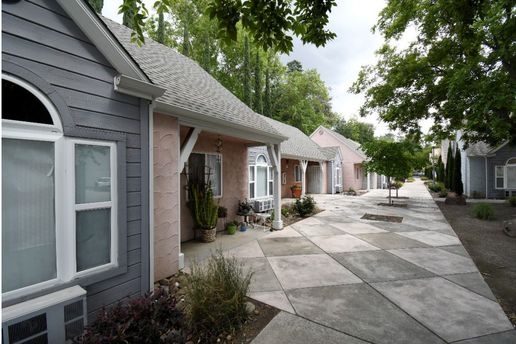
Walker Commons Apartments, 678 Buttonwillow Lane, Chico
