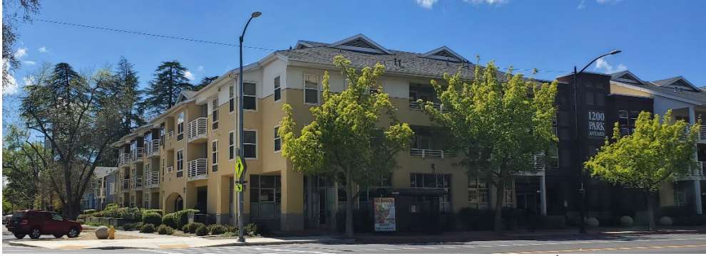
1200 Park Avenue Apts – Corner of Park Avenue and West 13 th Streets, Chico
