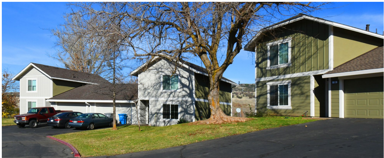
Evanswood Estates, Table Mountain Boulevard, Oroville - new exteriors.
