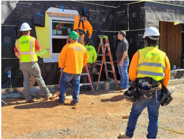
Window waterproofing coordination
