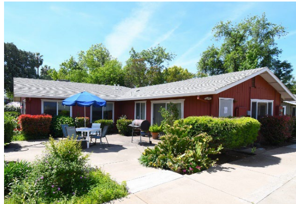
Community Building prior to improvements
