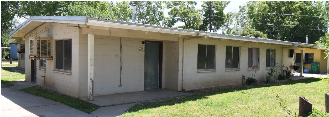
Unrenovated 1980's era Concrete-block Unit
