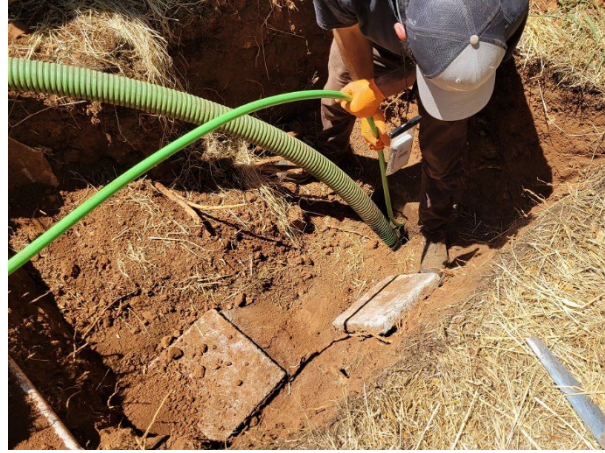
Septic leach line investigation
