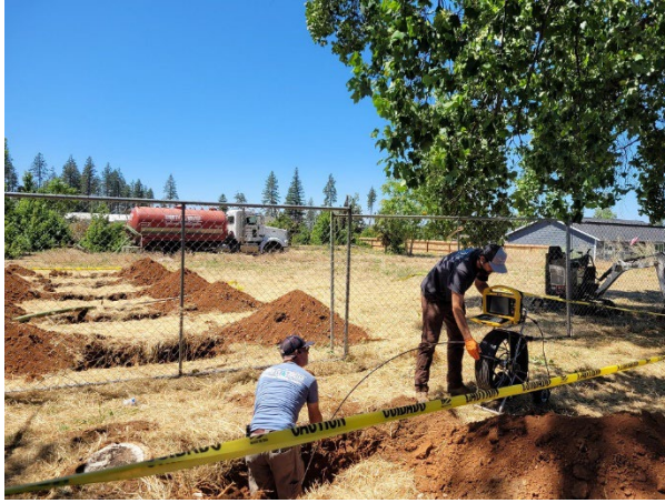
Septic leach line investigation
