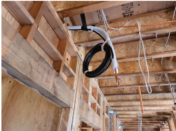
HVAC rough-in underway
