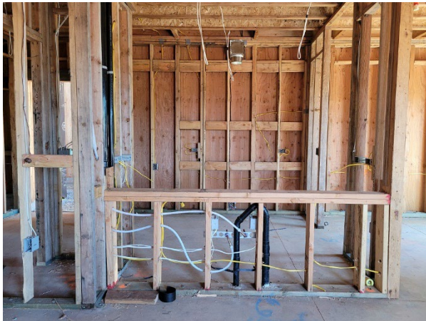
Plumbing and electrical rough-in complete
