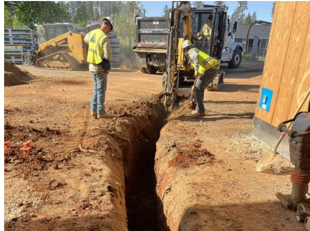
Installation of underground utilities
