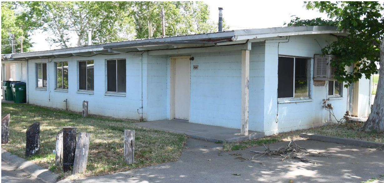
Unrenovated 1980's era Concrete-block Unit
