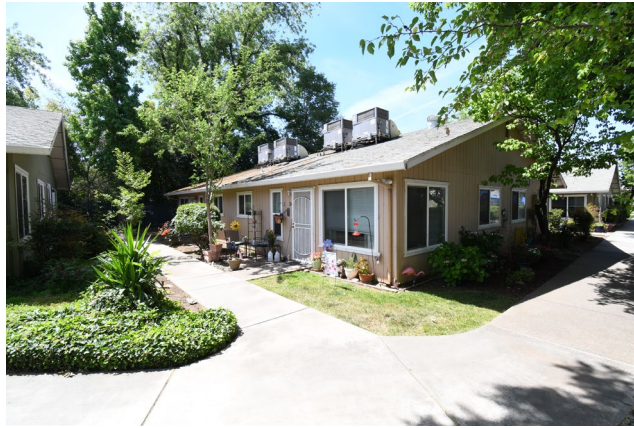
Park Place Apartments, 2105 Park Avenue, Oroville
