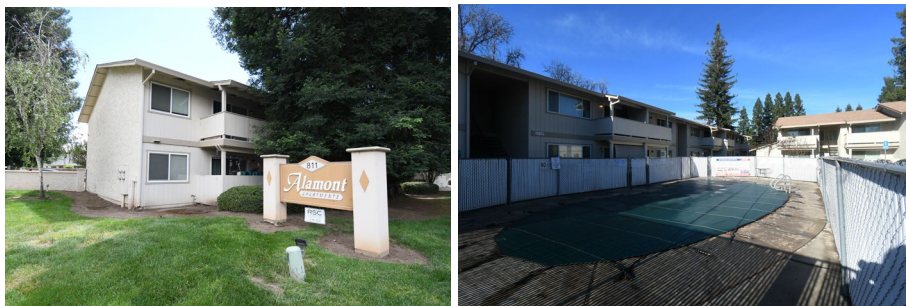
Alamont Apartments, 811 West East Avenue, Chico
