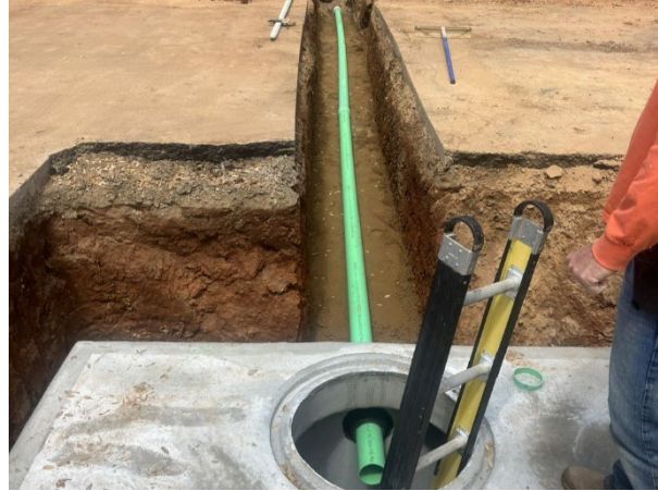
Installation of the new septic tank
