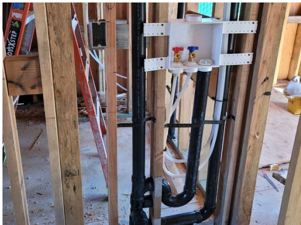
Rough plumbing installation complete
