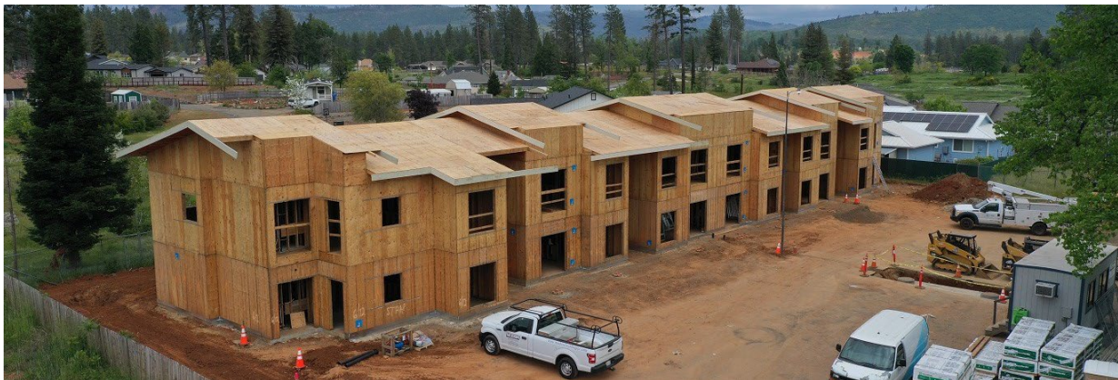
Aerial photo of construction progress
