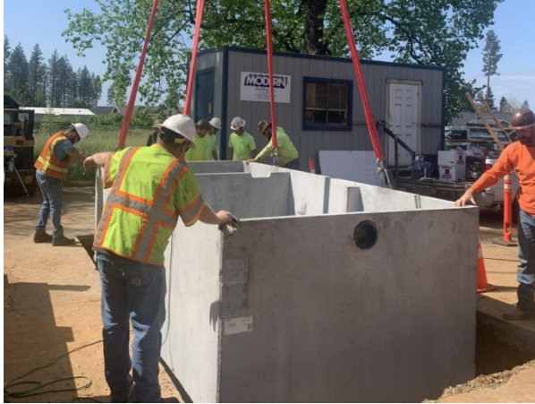
Installation of the new septic tank
