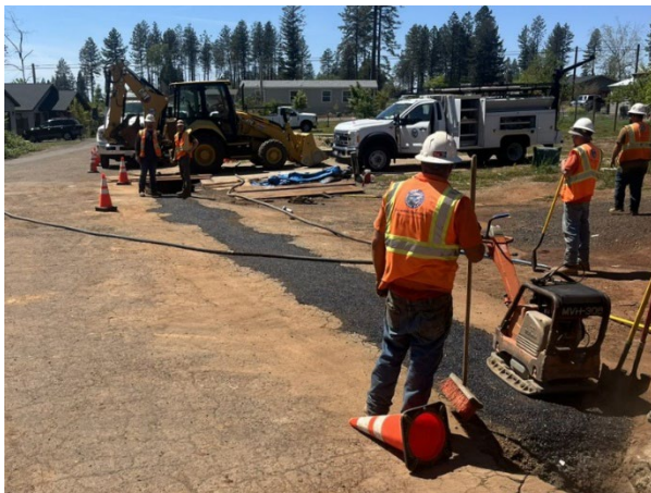
Installation of off-site utilities
