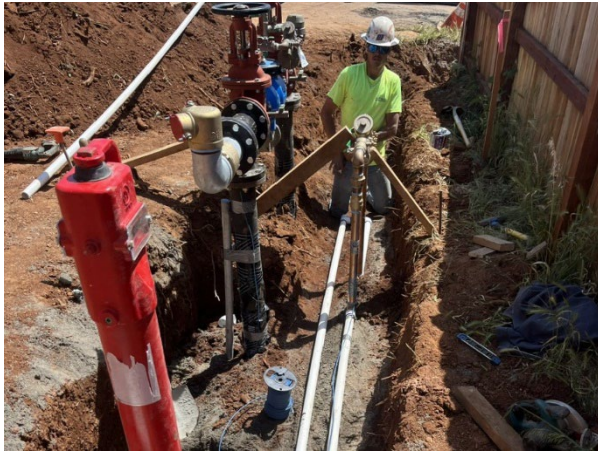
Installation of underground utilities
