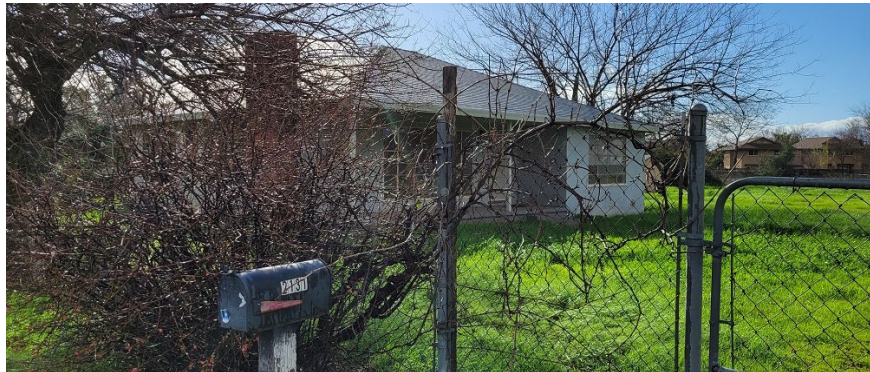
Project site and structure slated for demolition
