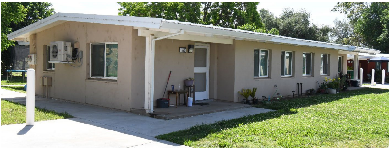
Renovated 1980’s era Concrete Block Housing
