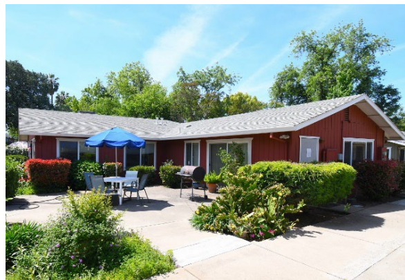
Community Building prior to improvements
