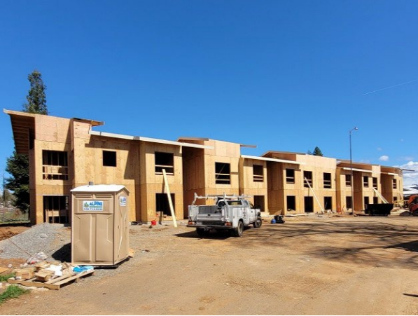
Rough framing nearly complete
