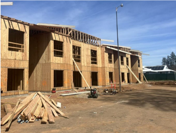
Pre-fabricated roof truss placement in process
