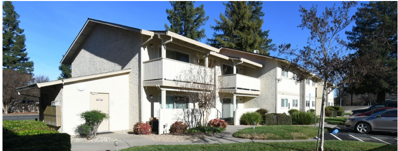
Alamont Apartments, 811 West East Avenue, Chico
