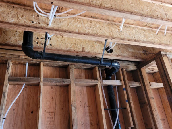
Rough plumbing installation in process
