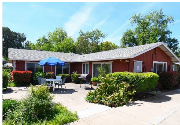
Community Building prior to improvements
