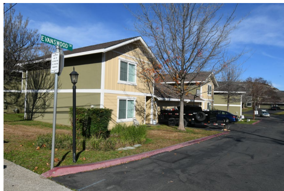
Evanswood Estates, Table Mountain Boulevard, Oroville - new exteriors.
