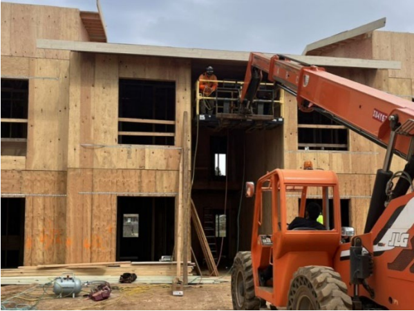
Installation of plywood wall sheathing
