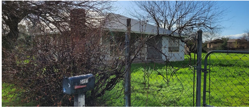
Project site and structure slated for demolition
