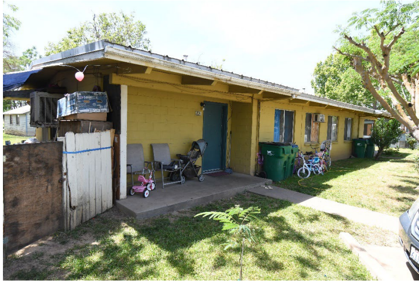
Unrenovated 1980's era Concrete-block Unit
