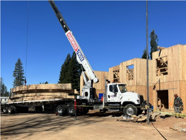
Pre-fabricated roof truss placement in process
