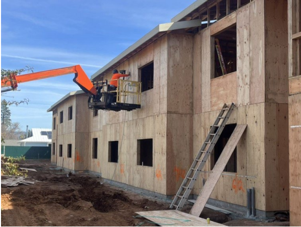
Installation of plywood wall sheathing
