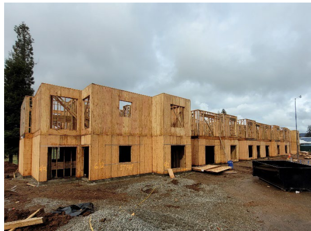
Second floor framing in process
