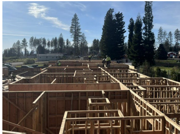
First floor framing in process
