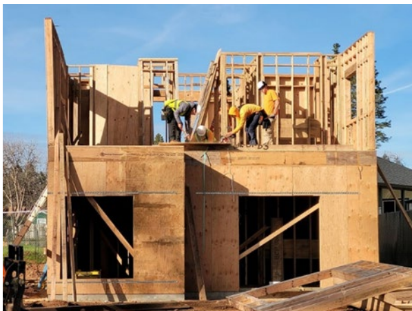
Second floor framing in process
