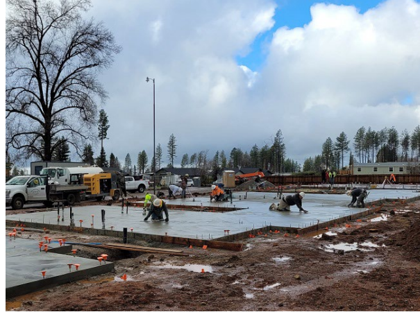
Concrete slab placement in process
