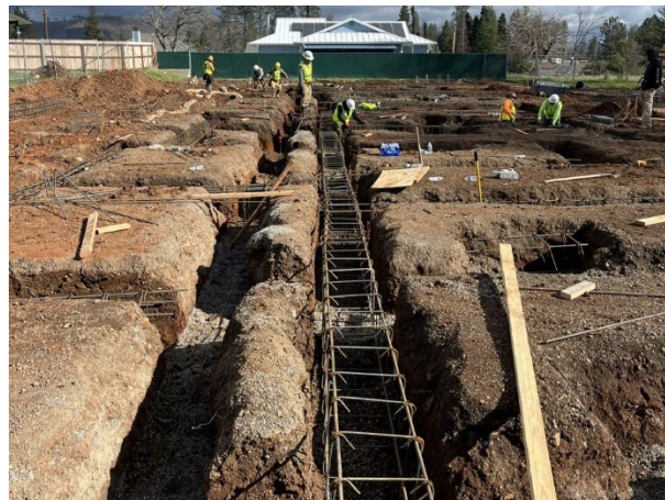
Footings excavated and rebar installation in process
