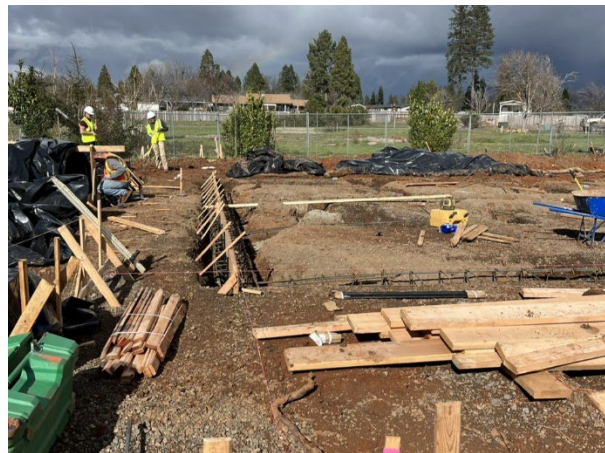
Foundation formwork installation in process
