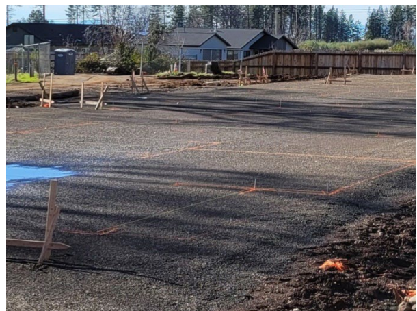
Completed Building Pad with Building Layout staked
