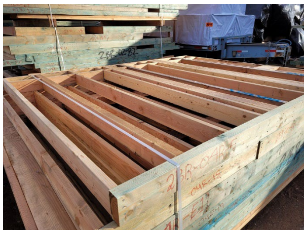
Pre-Fabricated Wall Panels stored on-site
