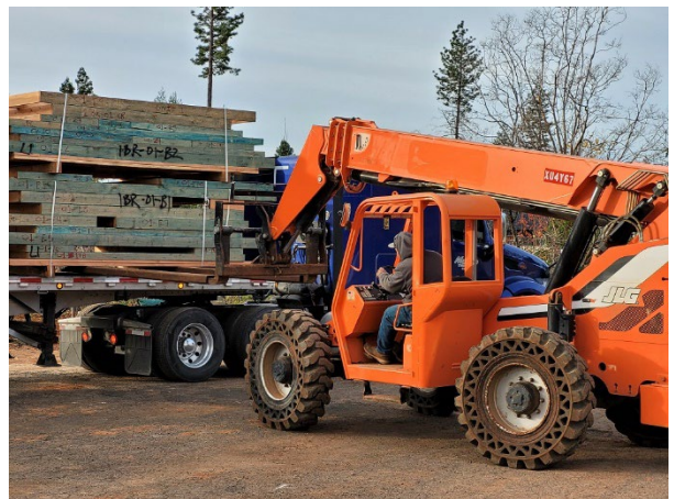
Delivery of Pre-Fabricated Wall Panels
