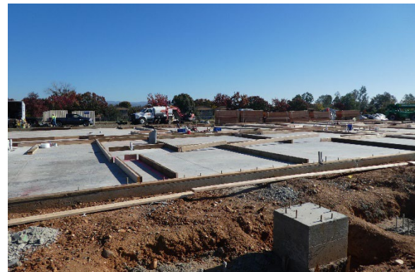
... to concrete slab on grade, ready to frame.
