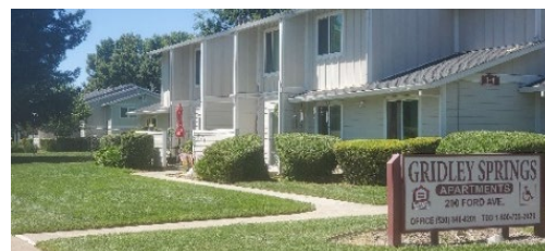
Gridley Springs I Apartments, Ford Avenue
