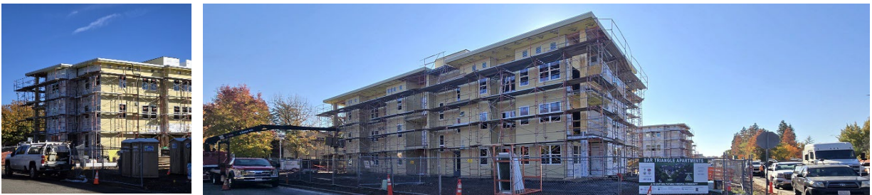
Bar Triangle Apartments, 2225 Bar Triangle Street, Chico – Framing underway
