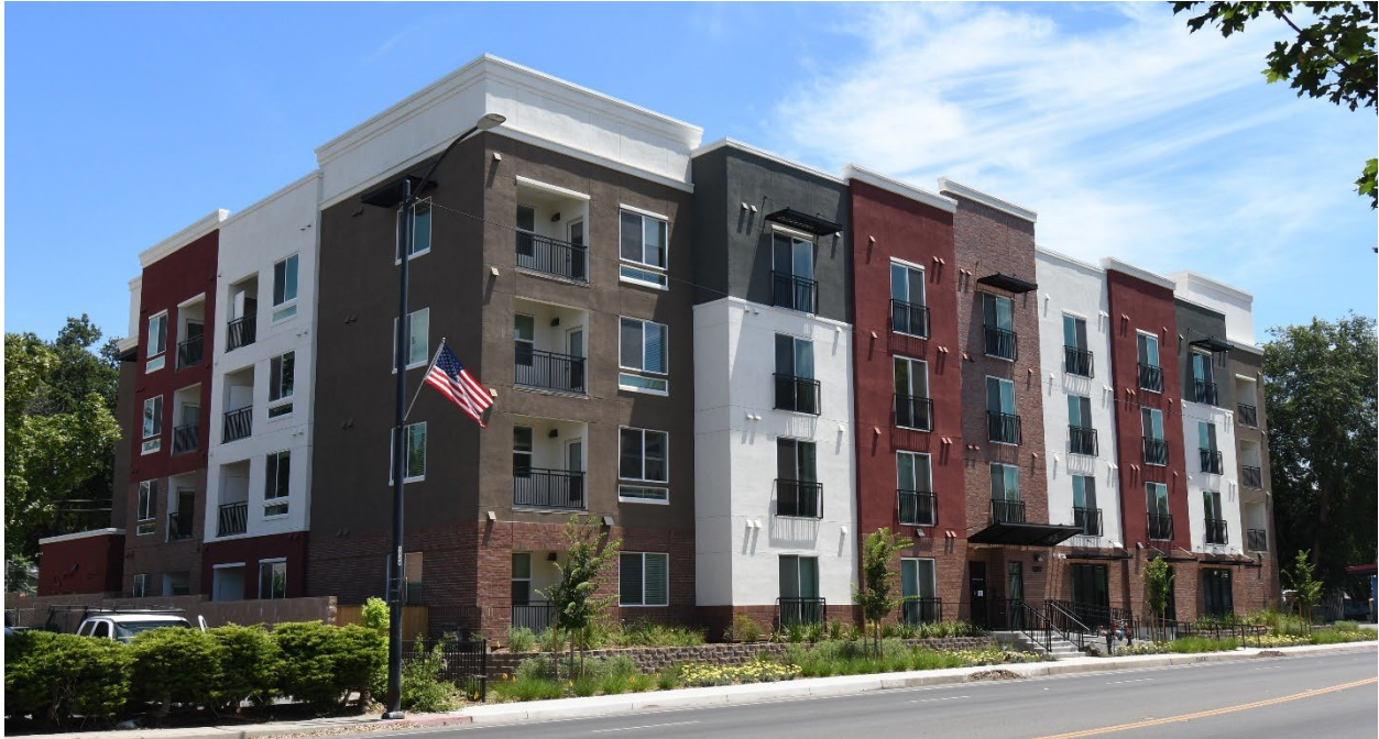
Park Avenue Apartments, 1297 Park Avenue, Chico
