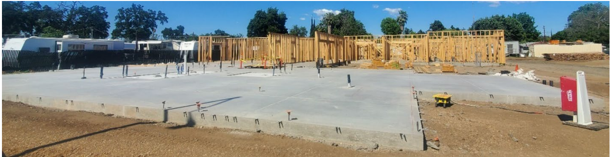
Oleander Community Housing Apartments, 2324 Esplanade, Chico – Framing underway
