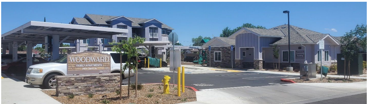
Woodward Family Apartments, 207 East Swift Street, Orland
