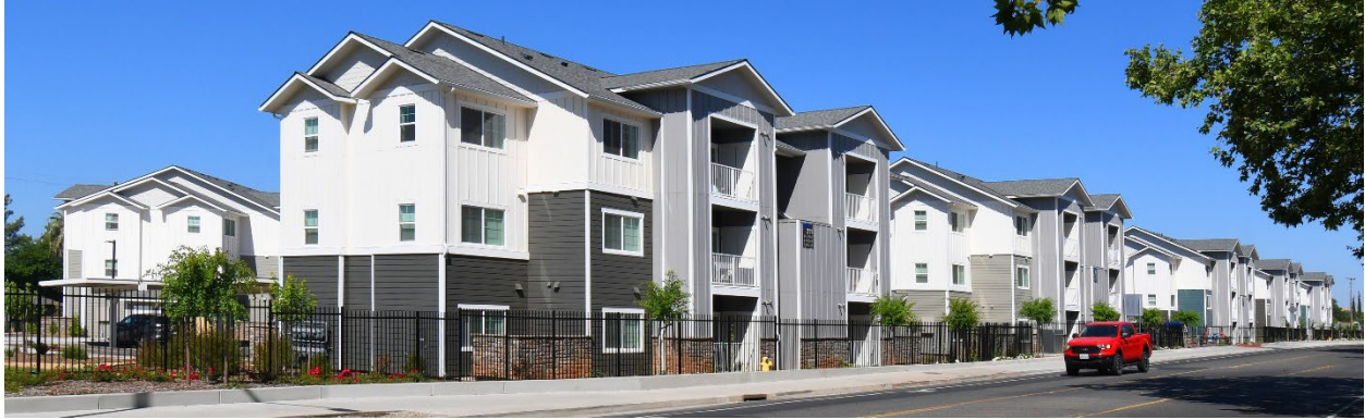
Riverbend Apartments I & II, Nelson and Table Mountain Boulevards, Oroville
