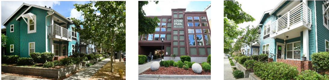
1200 Park Avenue Apartments, 1200 Park Avenue, Chico
