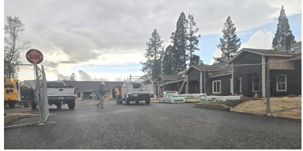
Northwind Senior Apartments, 6983 Pentz Road Framing is complete
