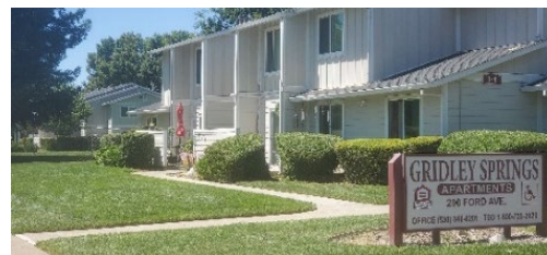
Gridley Springs I Apartments, Ford Avenue
