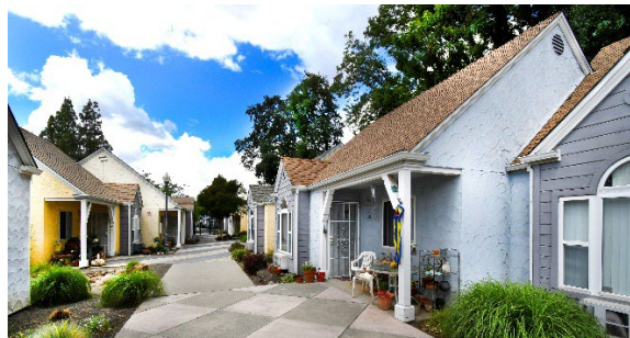
Walker Commons Apartments, Buttonwillow Lane, Chico
