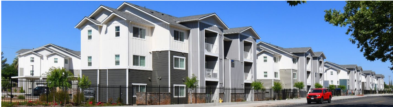
Riverbend Apartments I & II, Nelson and Table Mountain Boulevards, Oroville
