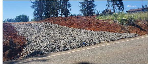
Northwind Senior Apartments, 6983 Pentz Road Sitework has begun
