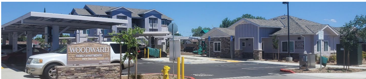
Woodward Family Apartments, 207 East Swift Street, Orland
