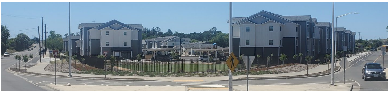
Riverbend Apartments I & II, Nelson and Table Mountain Boulevards, Oroville
