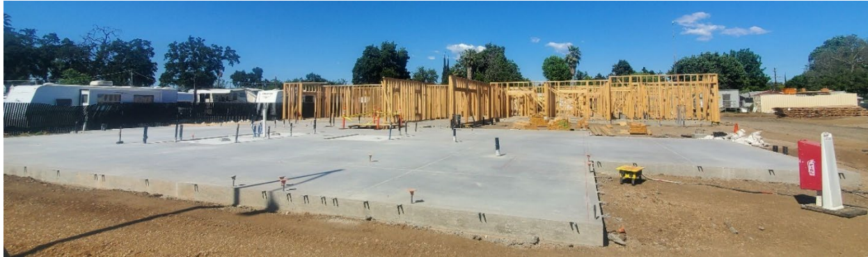
Oleander Community Housing Apartments, 2324 Esplanade, Chico, Framing underway
