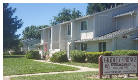
Gridley Springs I Apartments, Ford Avenue
