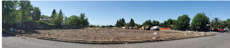
Bar Triangle Apartments, 2225 Bar Triangle Street, Chico – Site is cleared
