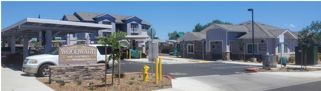
Woodward Family Apartments, 207 East Swift Street, Orland
