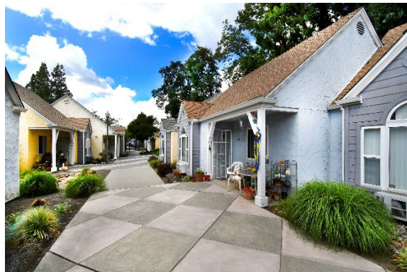
Walker Commons Apartments, Buttonwillow Lane, Chico
