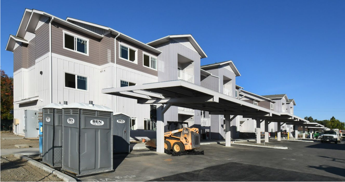
Woodward Family Apartments, 263 Swift Street, Orland
