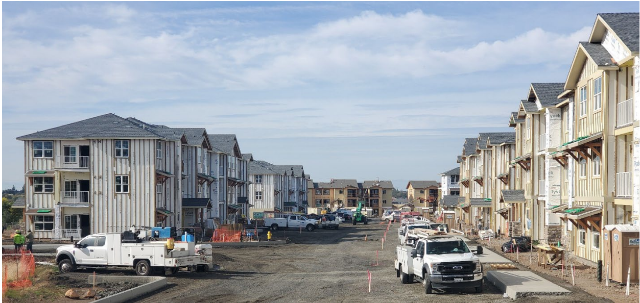
Deer Creek Apartments I & II, Highway 32, Chico
