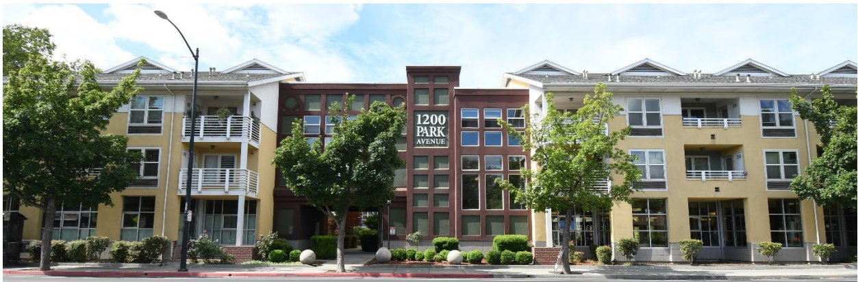
1200 Park Avenue Apartments, 1200 Park Avenue, Chico
