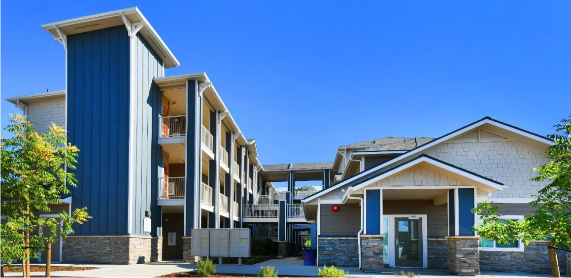
Mitchell Avenue Apartments II, Mitchell Avenue, Oroville
