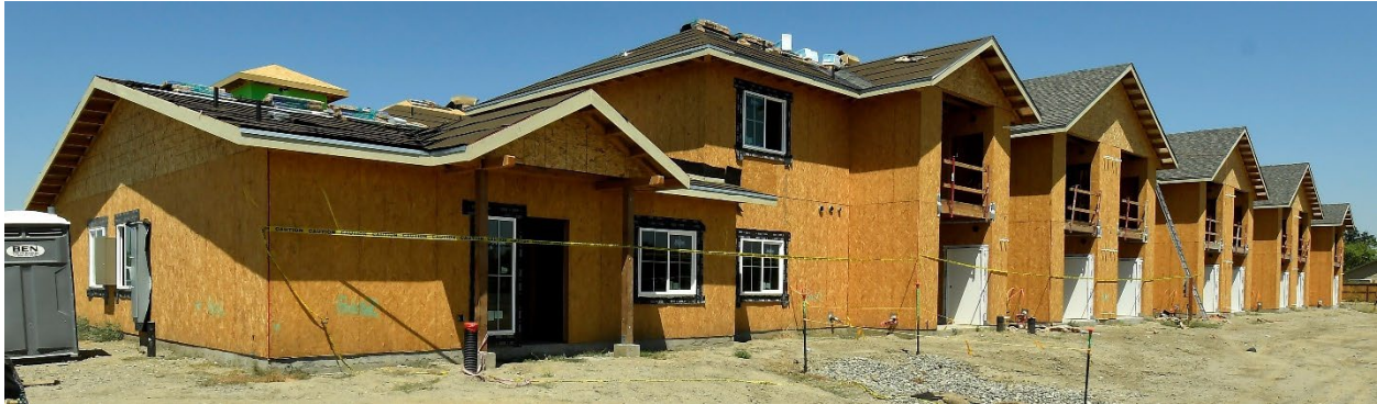
Liberty Bell Courtyard Apartments, North 6 th Street, Orland
